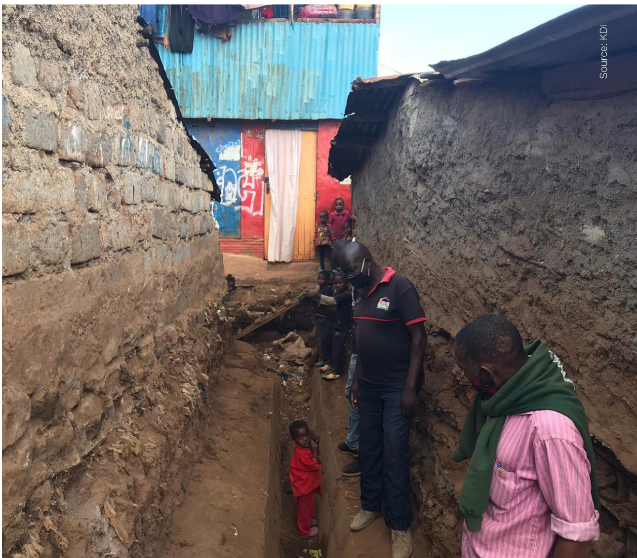
Figure 4: Example of open channel surface drain in Vuma neighbourhood, Kibera
